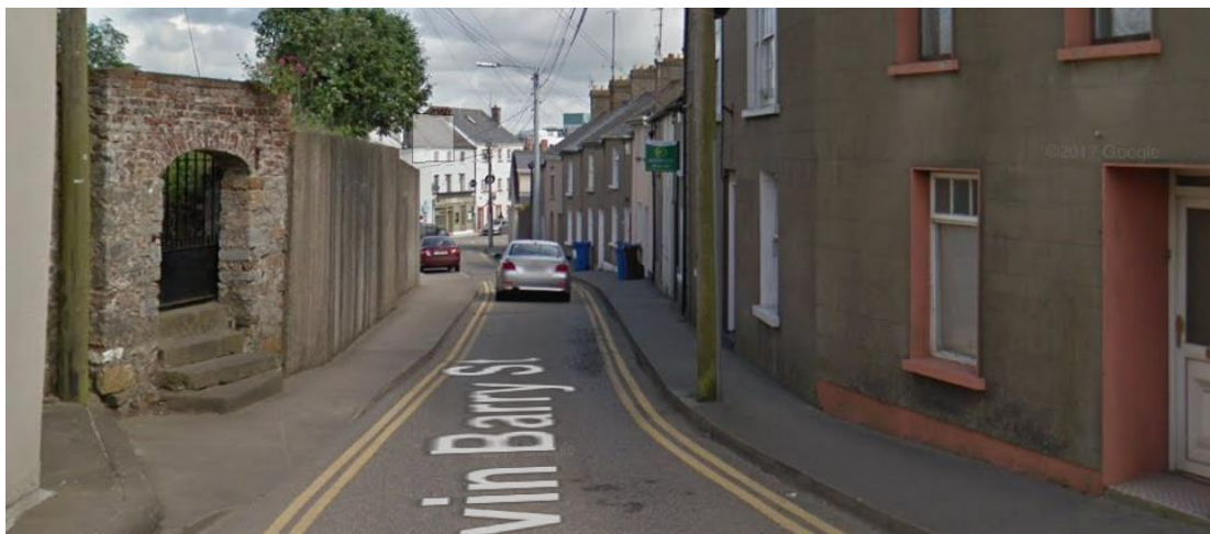
Plate 4.8 Kevin Barry Street – Note: narrow one-way street lined by high / medium density housing on one side.
