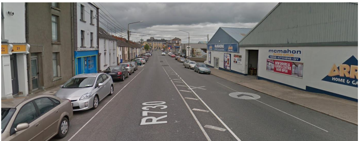
Figure 6 Trinity Street View in direction of Town Centre (North) from Proposed Access – one lane in each direction with on-street parking on both sides and ghost central median
