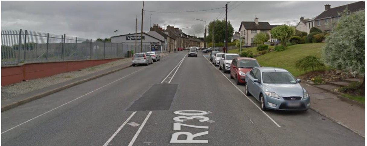
Figure 5 Trinity Street View South from Proposed Access – note one lane in each direction with on-street parking on both sides and ghost central median
